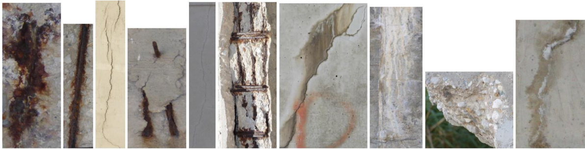
Figure 37 : CODEBRIM dataset examples of images with cracking, spalling, exposed rebars, corrosion.
