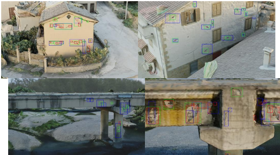
Figure 38: Some examples of semi-synthetic images with bounding boxes annotation of damages (different colours mark different type of damages)
