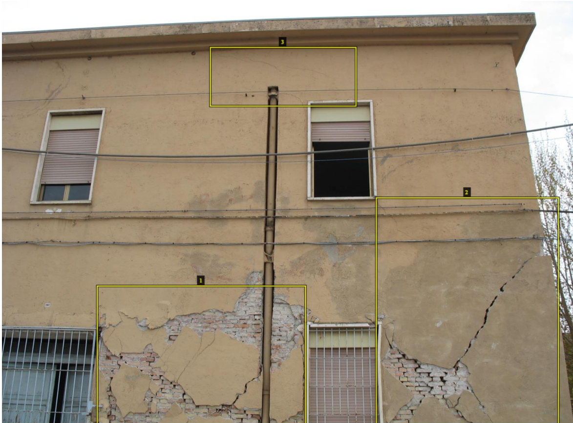
Figure 20: Example of an annotated image belonging to EUCENTRE'S dataset (L'Aquila 2009 event, shear damage on unreinforced masonry piers and spandrels)
